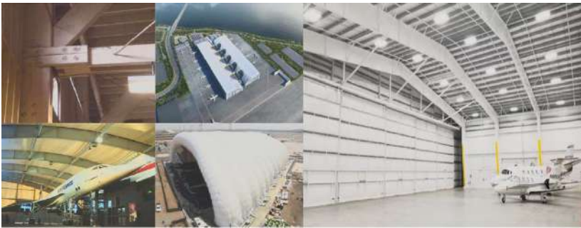
Fig. 1. Wooden structure hangar, concrete structure hangar, metal structure hangar, inflatable hangar, steel structure hangar
